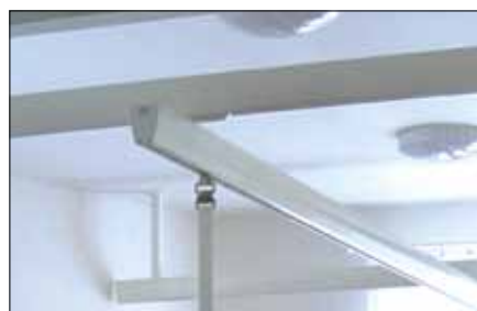
Traverse system - provides the opportunity to move across the room's entire surface.
